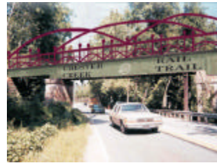
"Graffiti Bridge" over Pennell Road, after conversion to a trail
